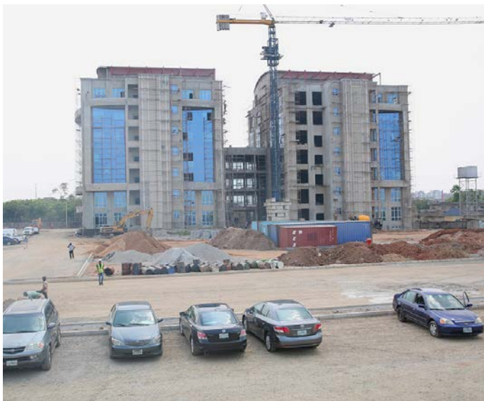
New IHVN building
